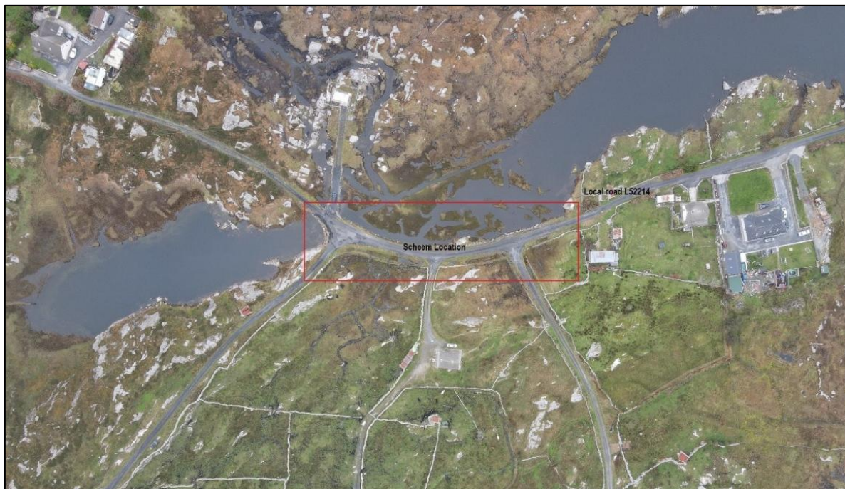
Figure 5.2 Aerial view. March 2025
